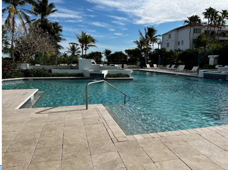
Pool/Spa Equipment and Heaters - 2028
