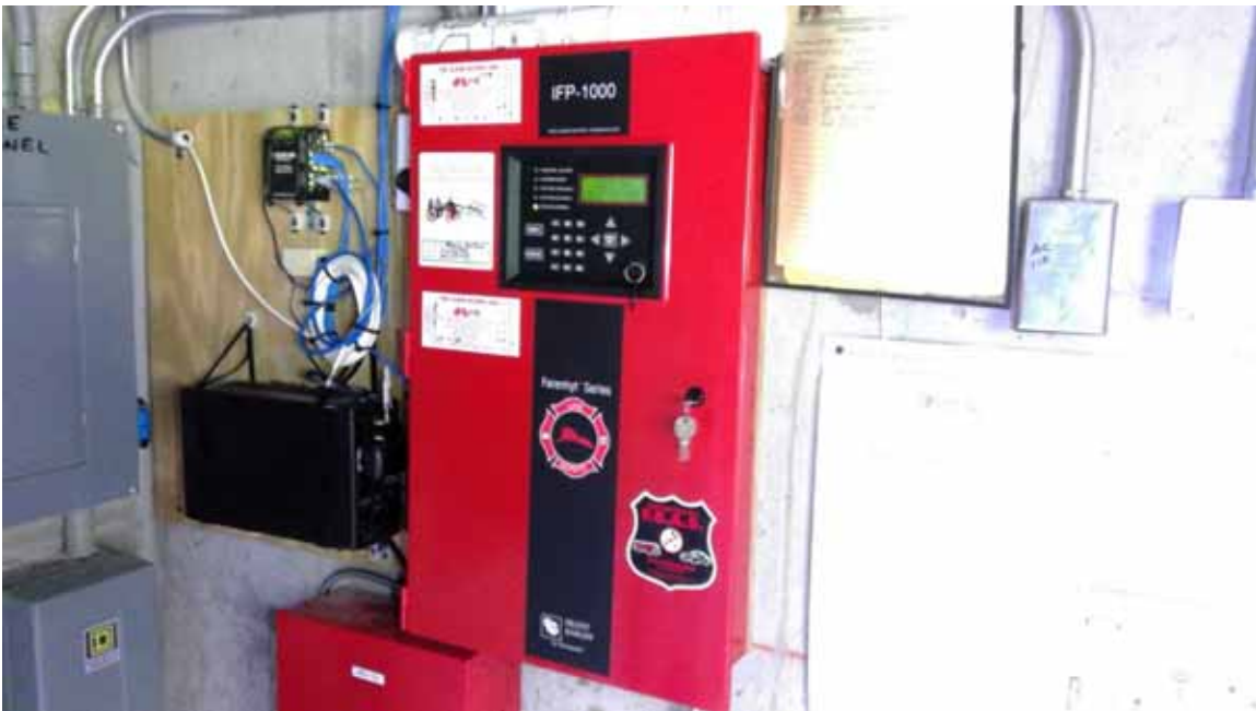
Condo Bldg Fire Alarm Panel
