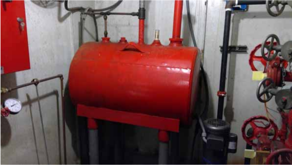
Fire Pump Diesel Tank
