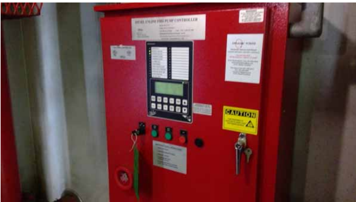
Fire Pump Controller
